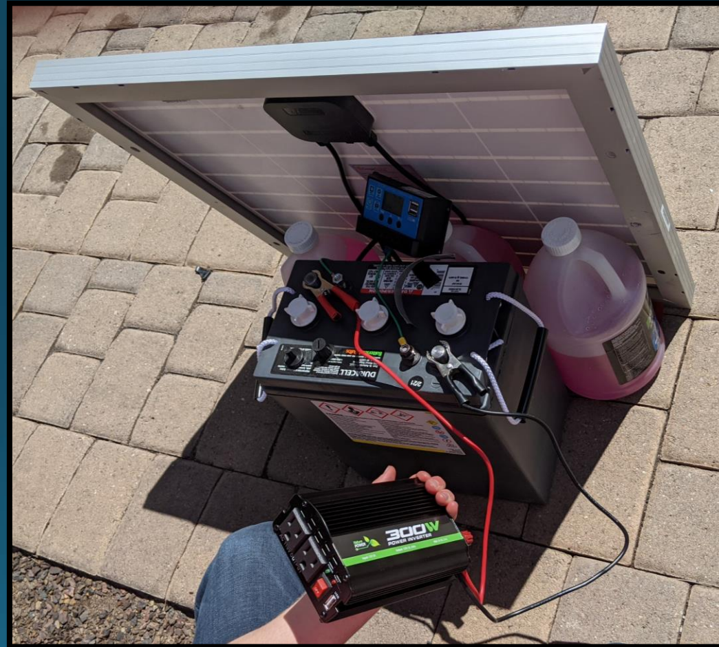
Figure 13: Solar Panel with battery and inverter
